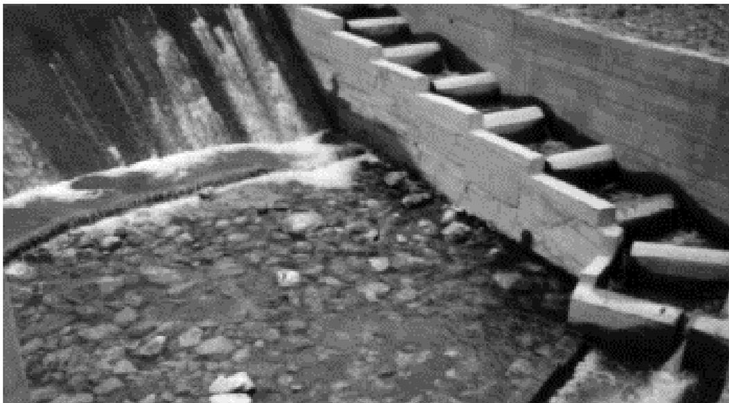
**Photo 7.14: Fishpass with vertical slots**
