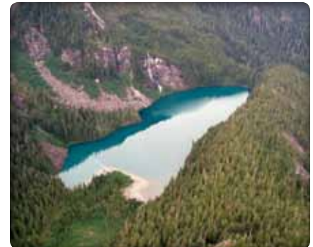
At 865 meters above the turbine, Tyson Lake acts as a storage reservoir. The lake is 60 meters deep and offers plenty of reserve.
