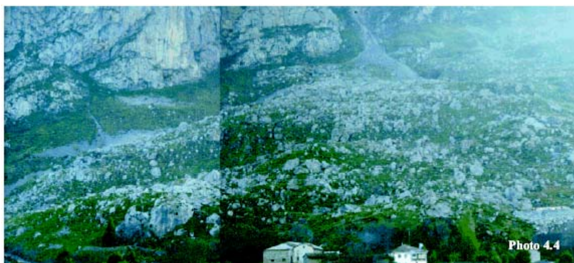
Photo 4-4 A view of the Cordiñanes colluvium, under which the tunnel runs
