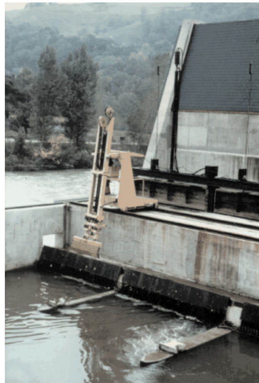
Photo 5.10: Telescopic hydraulic cylinders
