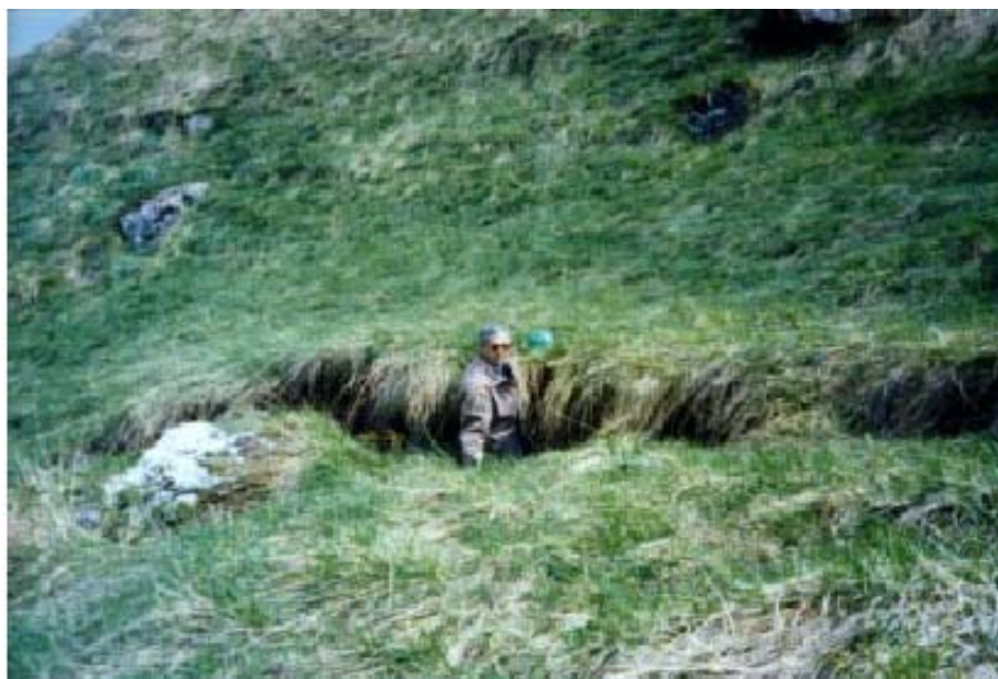
Photo 4-3 One of the existing sliding scarps before the beginning of the works
