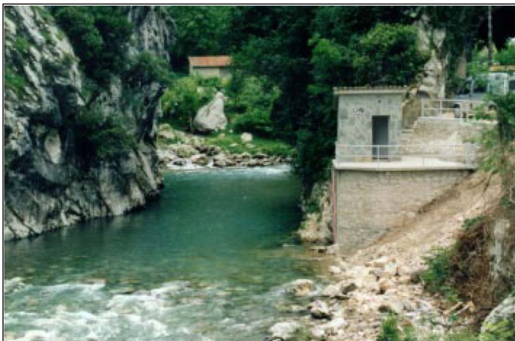
Photo 3-1 Gauging station in a river
