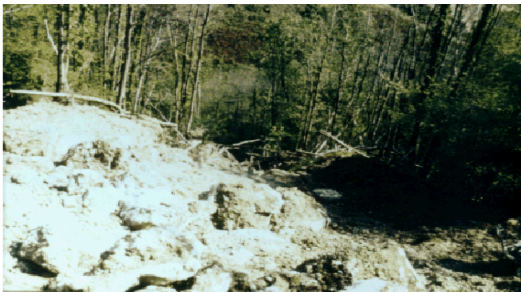
Photo 4-10 Weir undermined by seepage
