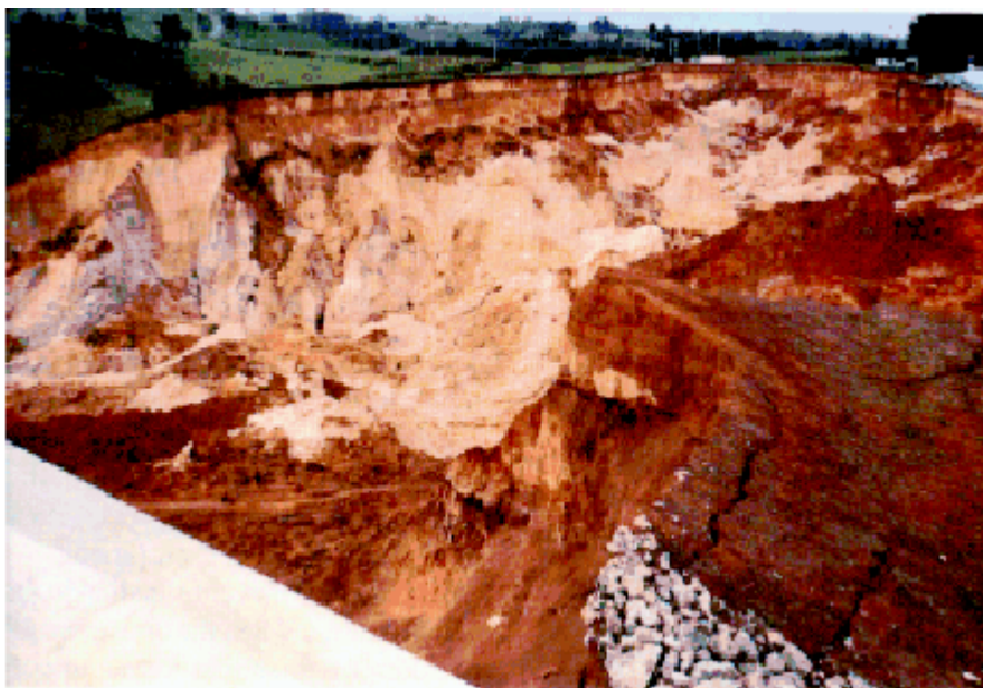
Photo 4-8 The effects of failure
