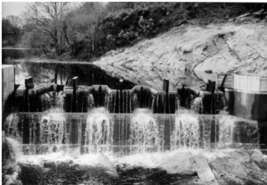
Photo 5.7: Hydroplus fusegates
