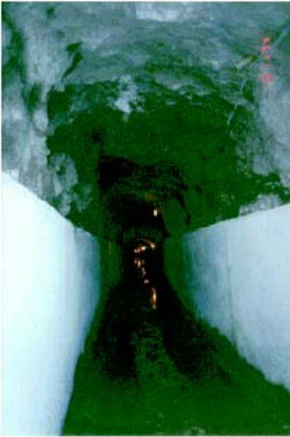
Photo 4-7 View of the tunnel lining
