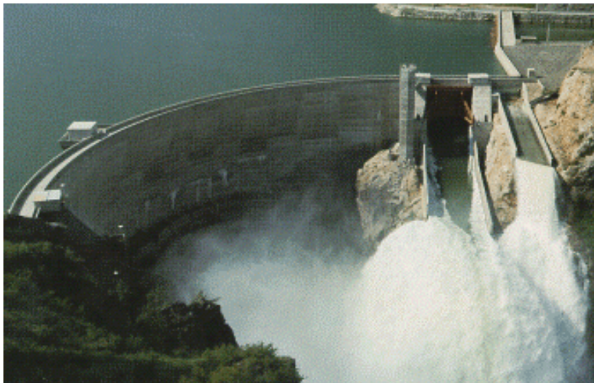
Photo 5.2: Example of an arch dam
