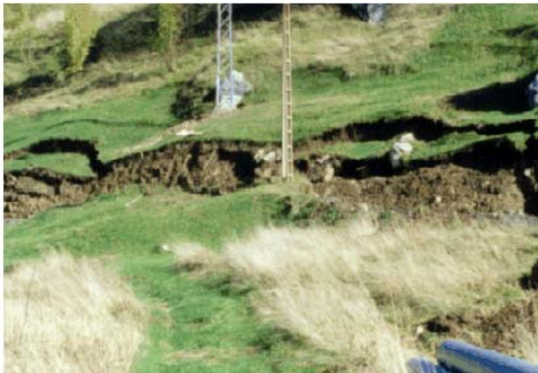
Photo 4-1 General view of the right-side slope
